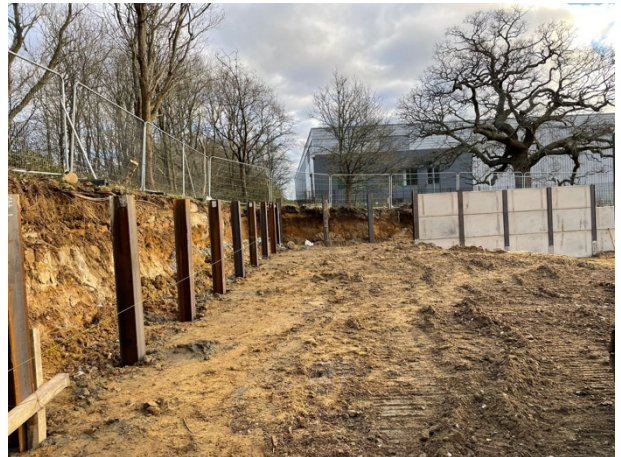
Figure 1: The site with part of the kingpost wall
